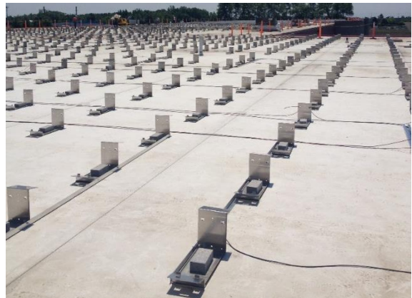
Fig. 2 - Supports Placed Prior to Ballasting
