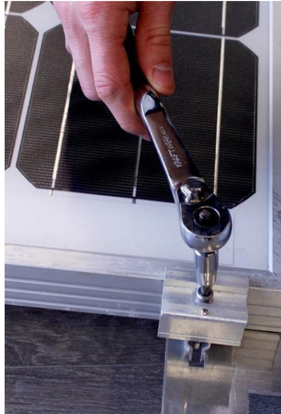
Fig. 14 - Use Torque Wrench
