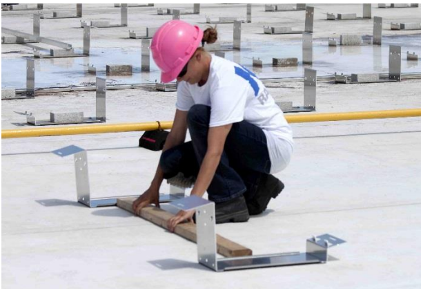
Fig. 1 – Use of Spacer Sticks to Aid Placement
